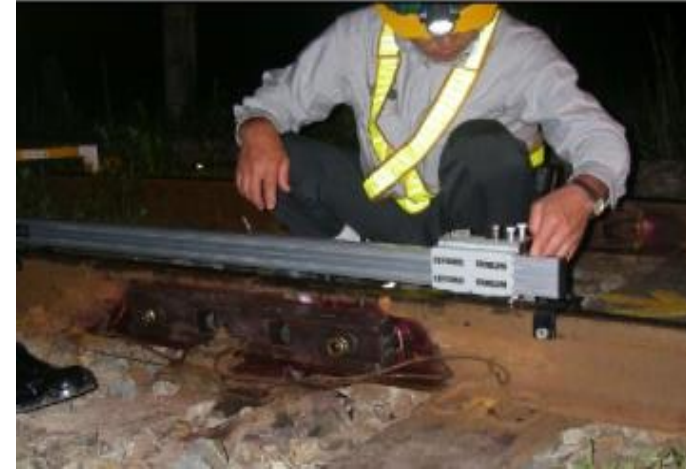
Measurement of surface roughness
